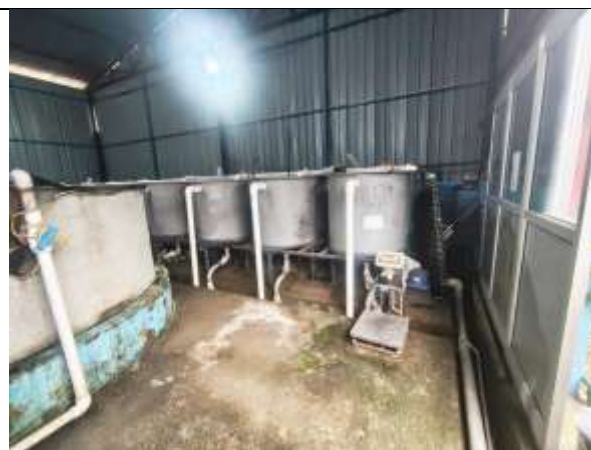
After cleaning inside RAS facility
