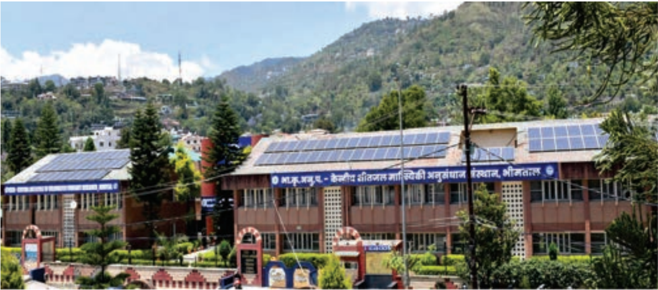
Main office building of ICAR-CICFR, Bhimtal
