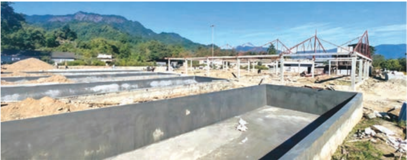
Hatchery and pond civil work in progress at NHPC, Dollungmukh, Lower Subansiri
