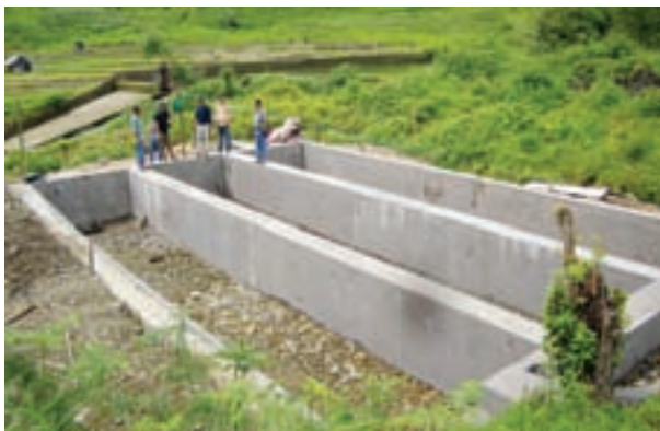
Construction of trout raceways at Dzuleke, Nagaland
