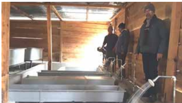
ICAR-DCFR financed trout hatchery being renovated in Shergaon Trout farm, Arunachal Pradesh
