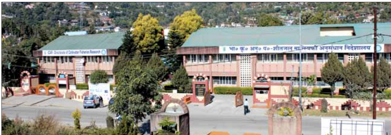
Main office building of ICAR-DCFR, Bhimtal
