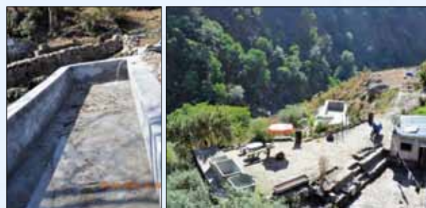
Construction of trout raceways at Pithoragarh district
